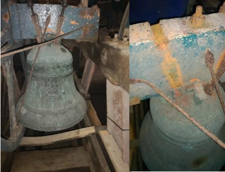
Corroded bell fittings
